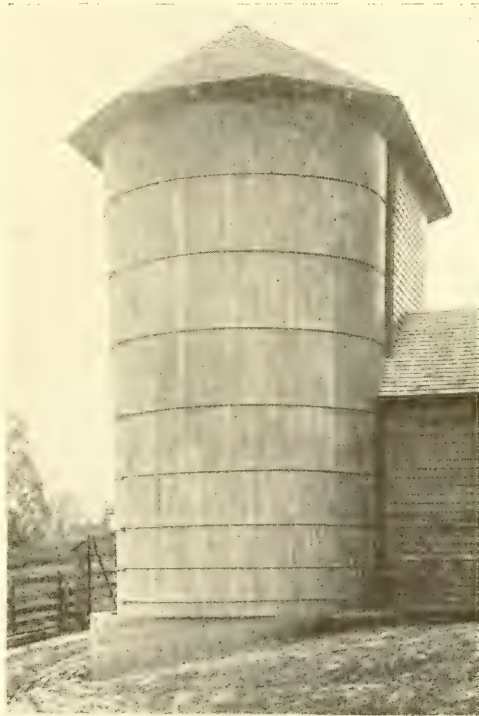
Wood Stave Silo Displaced by Wind —Photo by Courtesy of Virginia Agr. Exp. Station
